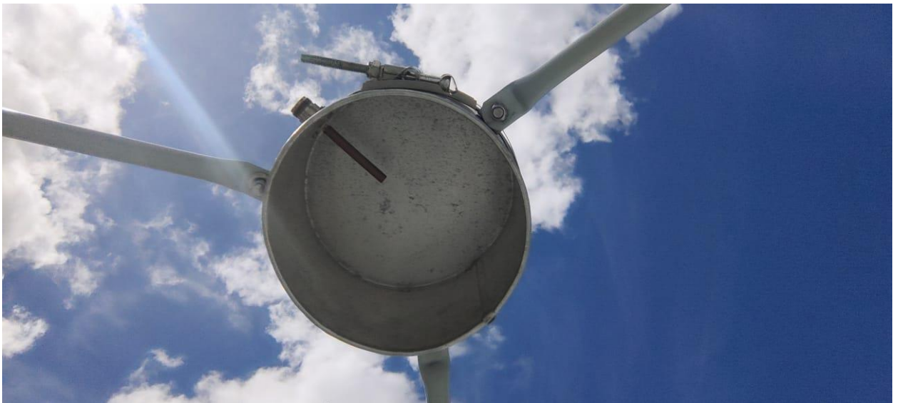
Antenna viewed from bottom with Monopole inside
